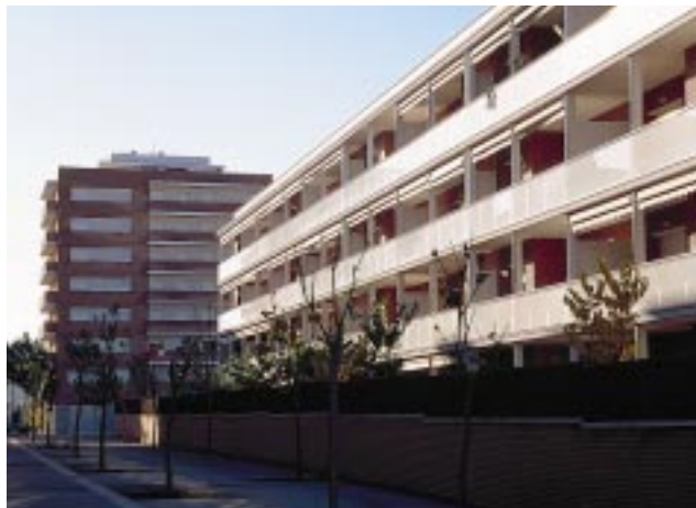
The heat plant run on biomass supplies heating and hot water to 250 dwellings in La Granja residential area, Molins de Rei.
