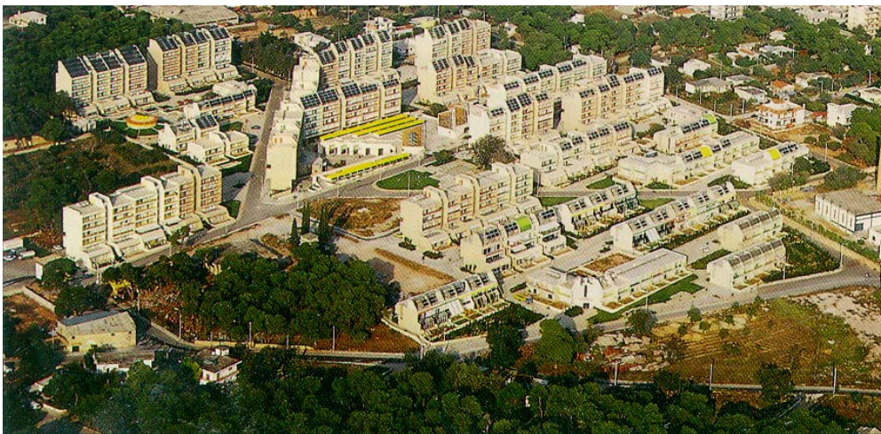
Figure 1: View of Solar Village in Pefki
